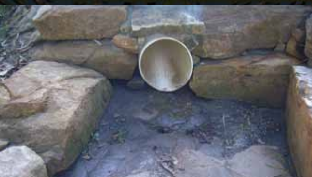
Stormwater pipe into sedimentation basin
