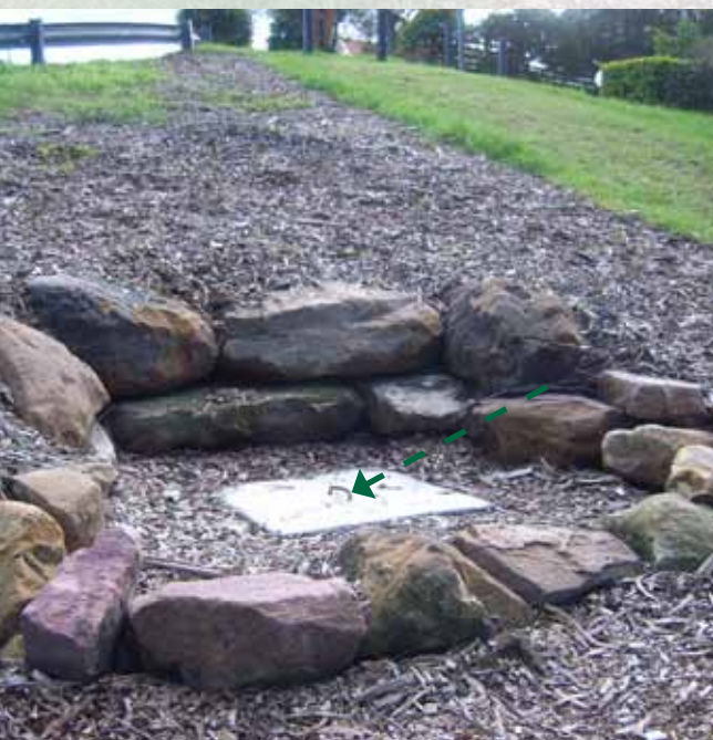
Headwall and junction pit (centre) of existing and new stormwater pipes
