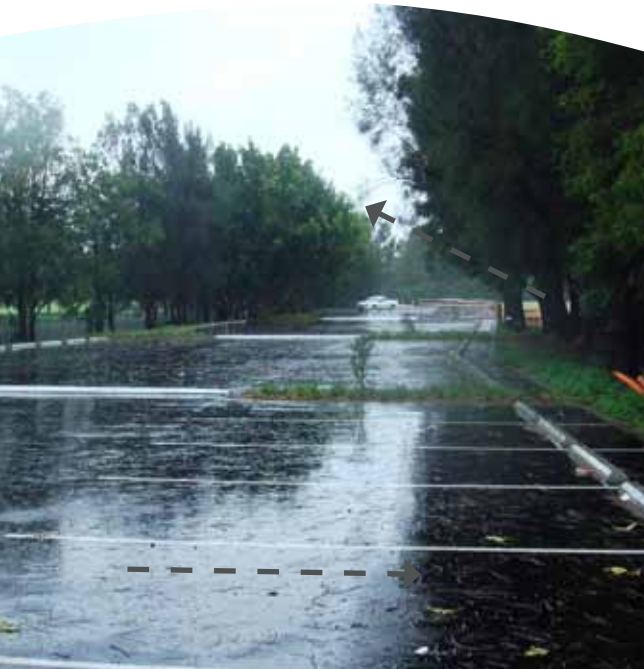
Mason Park car park (new surface) directing water flow to swales
