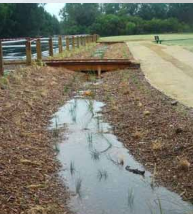
Vegetated swale with ponding during a storm event, 2010.
