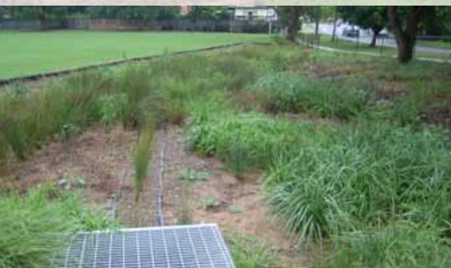
Stormwater outlet and the channel, 2010.
