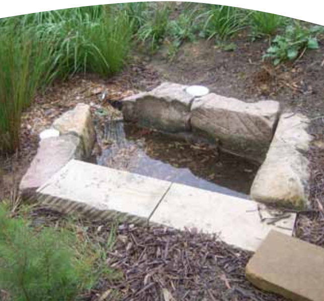
Rock sedimentation basin at entrance to the system
