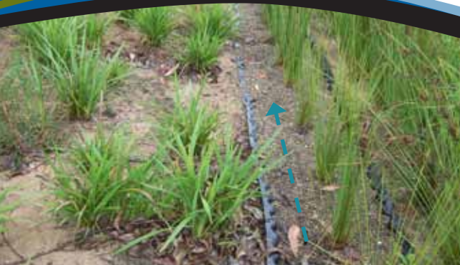
Flow dissipation channel filled with gravel
