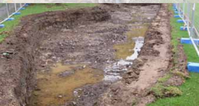
Excavation of the basin, 2009.
