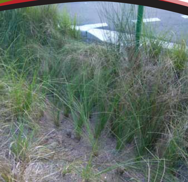
Rain garden at corner of Railway and Constitution Roads
