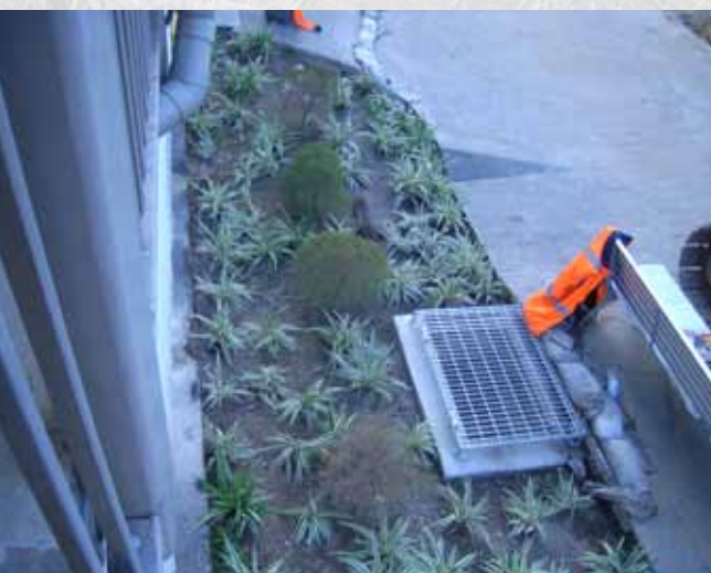
Rain garden (and stormwater outlet) at the railway station
