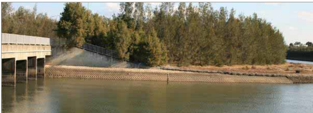
Figure 4-7. Grout mattress revetment
