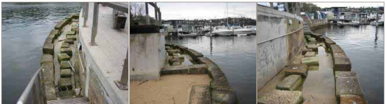
Figure 4-19. Pools that hold water at low tide created against existing seawall adjacent Spit Bridge, Mosman LGA.
