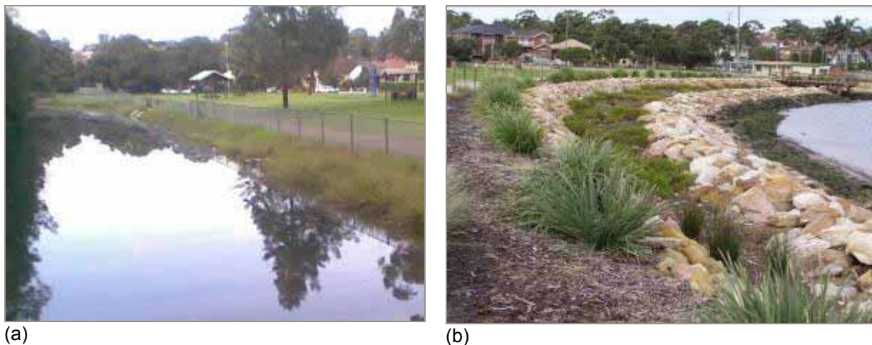
Figure 4-11. (a) King tide overtopping crest, Hawthorne Canal, Ashfield LGA (b) Seawall design that allows overtopping of high tides to inundate saltmarsh vegetation Claydon Reserve, Kogarah LGA
