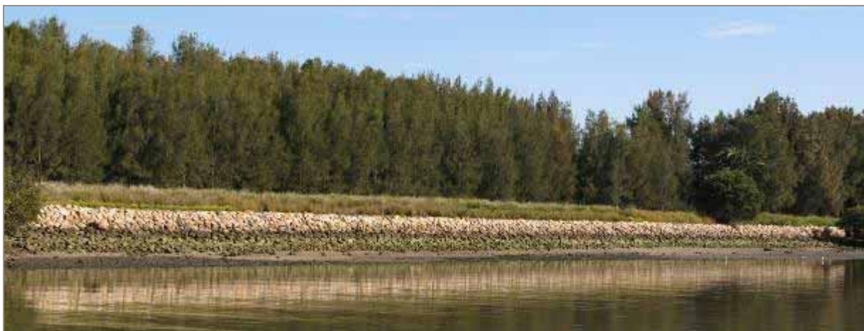
Figure 4-5. Sandstone rubble revetment
