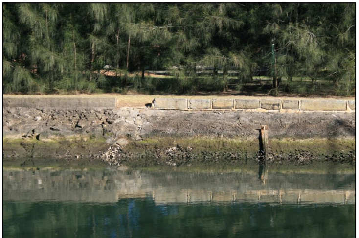
Photo 2 Transition of revetment into Hawthorne Canal.
