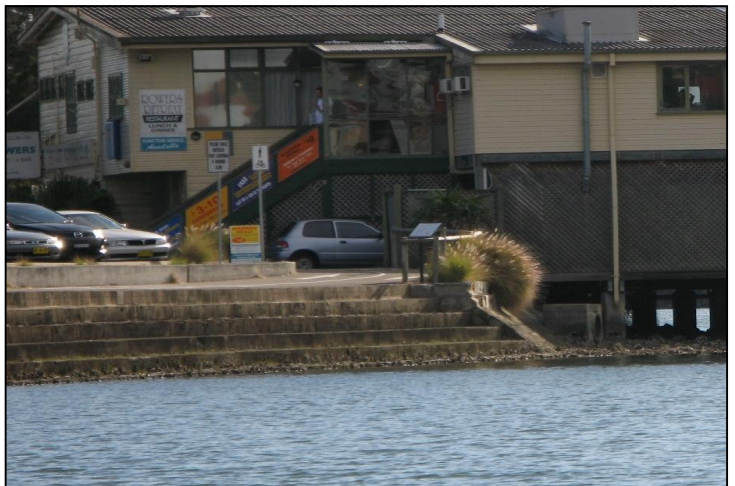
Photo 2 Sandstone sea stairs adjacent to the UTS Rowing Club house.
