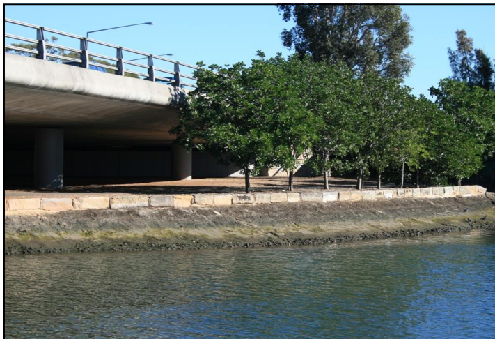
Photo 1 Typical section of revetment.
