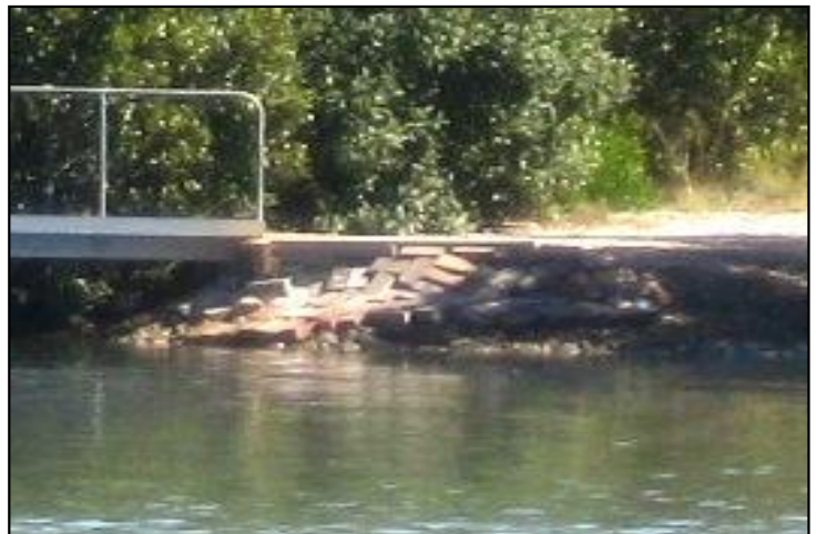
Photo 2 Collapse of blocks that form revetment.
