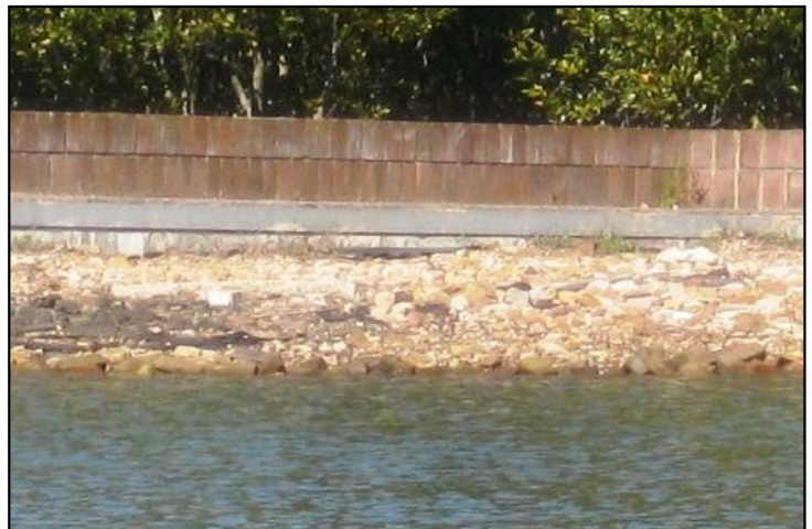
Photo 2 Failure of blocks exposing soil and undermining concrete slab on crest.
