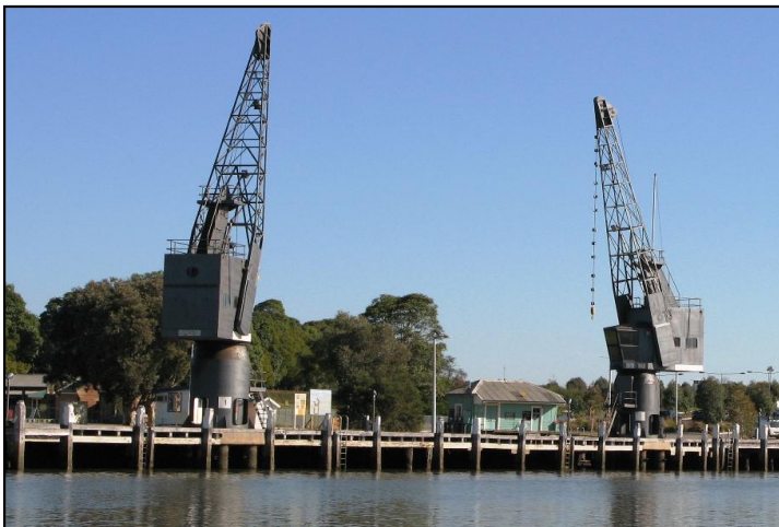
Photo 1 View of facility.
