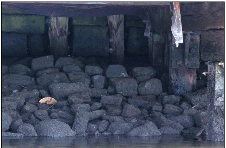
Photo 2 Timber piles, sandstone block seawall and rubble revetment beneath structure deck.
